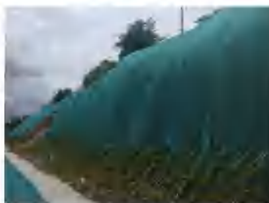
边坡临时苫盖
