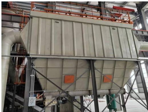
研磨包装废气布袋除尘
