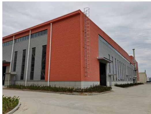
研磨废气排气筒
